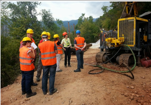
“Regular site visits by our environment and social teams ensuring the smooth running of all our monitoring programmes.” - Elizabeta Stoeva, Information Centre Administrator
